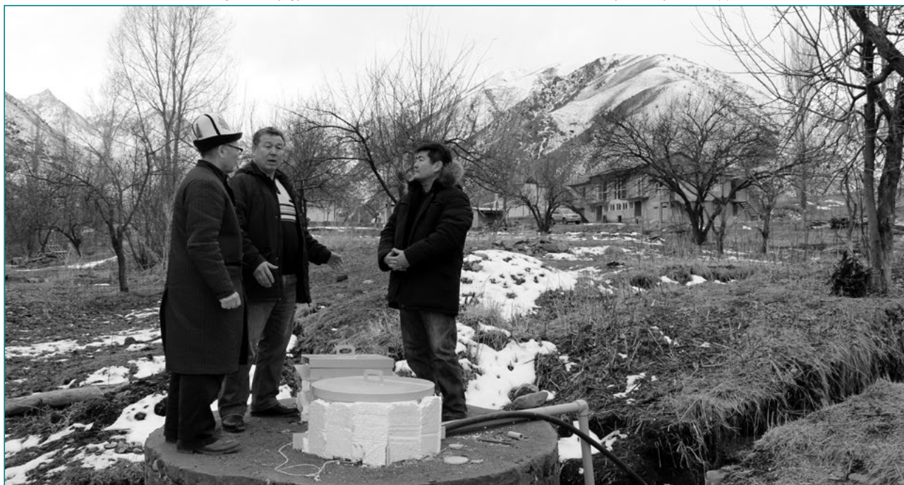
Figure 9 Eco-resort »Ak-Tilek« in the Chui region of Kyrgyzstan, which installed a wastewater treatment facility with KyrSEFF support
