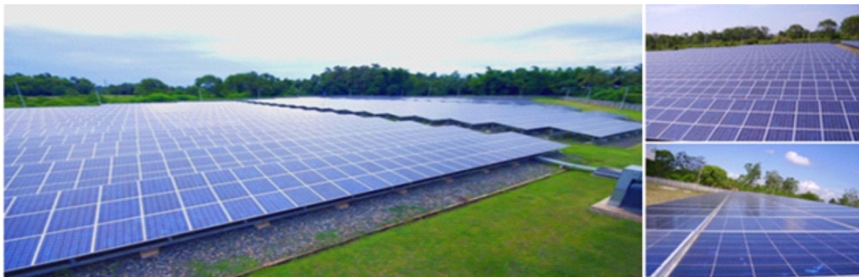
Figure 9. 1-MW Photovoltaic Power Plant, Barangay Indahag, Cagayan de Oro City, Philippines
