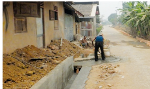
Figure 6.7 Building Permanent Ditch/Siring
