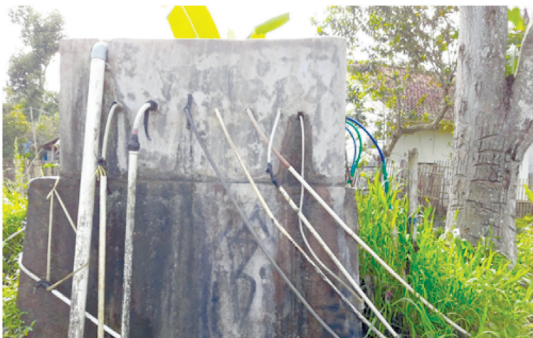
Gambar 2.3 Sistem Distribusi Air (Sistem Cacing)
