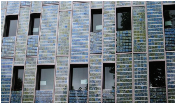
Figure 25: Colored PV panels on the Facade of a Building - La Cita Vita ( www.flickr.com/photos/la-citta-vita/5964294206/ ).
