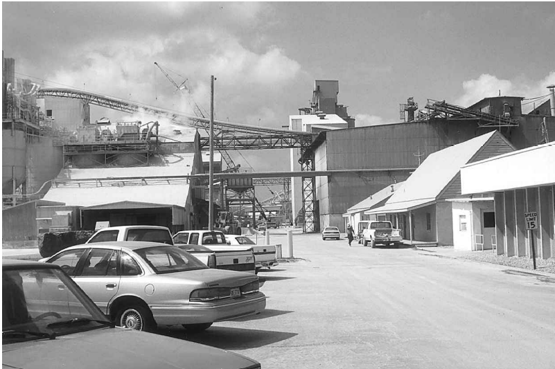
FIGS. 1 AND 2. Blue Circle Cement Plant, Calera, Alabama, 1999.
