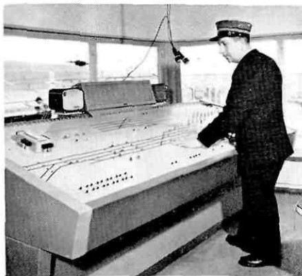
Up-to-date equipment and facilities characterize the Swiss railway network. Track and safety installations are of the highest order, resulting in an efficiency and a safety record which can compare with the best anywhere else in the world.
