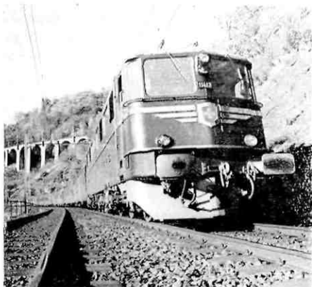
It costs several times as much to lay a track in mountainous districts as on the flat, but fares on the Swiss railways are no higher on the mountain routes than elsewhere. One of the most expensive items has been the construction of tunnels.
