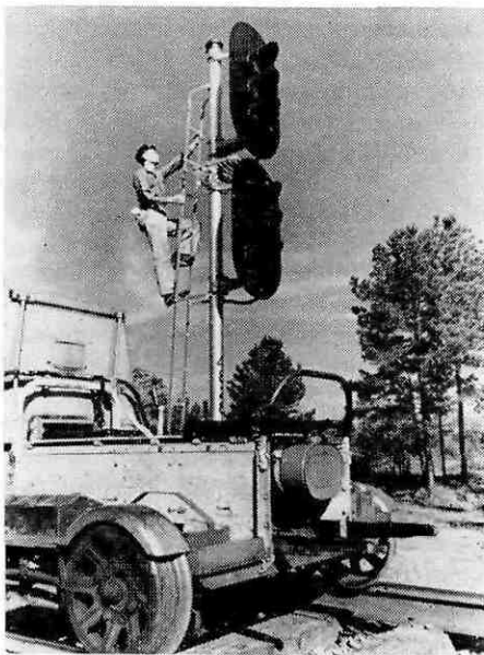
Constant and careful signal inspection contributes towards the safety of rail travel. US railroad labor organizations have fought for and helped to bring about every safety regulation and device now taken for granted, including the signal system now in use (Seaboard Air Line Railroad Co)
