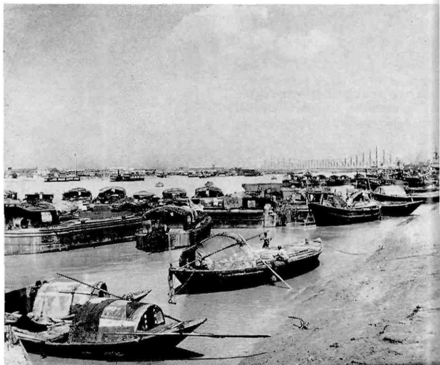
A scene on the Hoogly River with a distant view of the port of Calcutta. The unsuitable nature of the river for deep-laden craft has recently led the Indian government to consider the construction of an auxiliary deep-sea port approximately sixty miles farther down the river at Haldia
