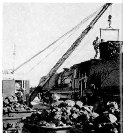
African railway workers help in re-cooling railway engine at a depot in Southern Rhodesia. The method being used, however, is purely temporary arrangement and a new electric loader will shortly be placed in service (Photo: Rhodesian Federal Information Department)
