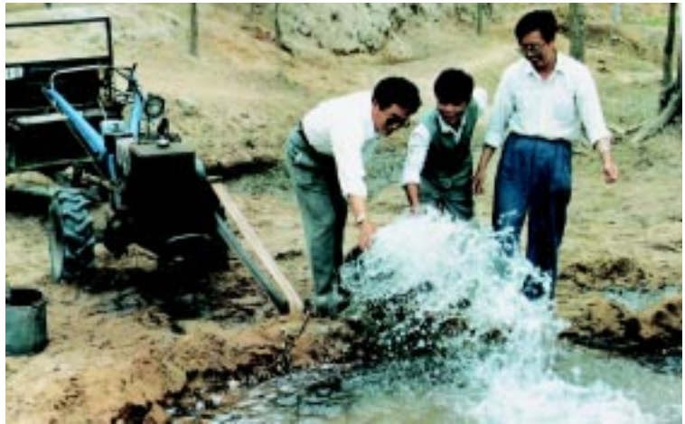
A pump extracts ground water close to the surface
