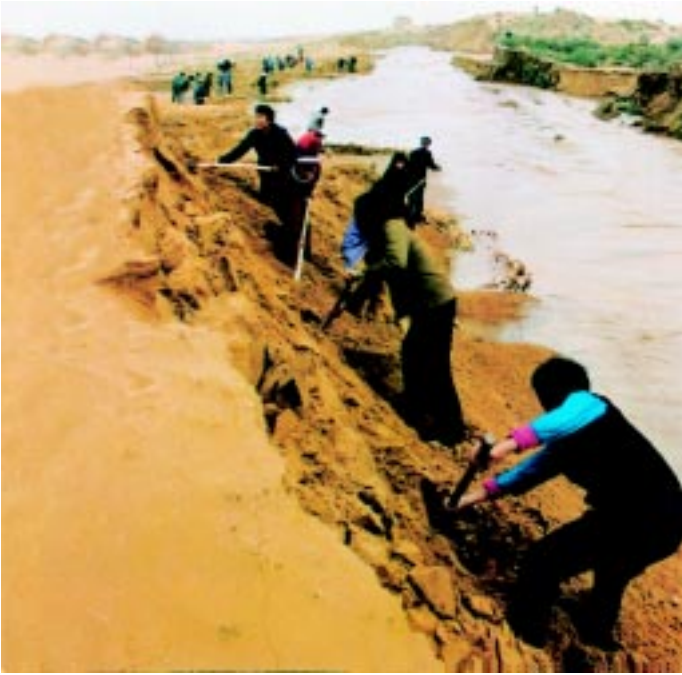
Levelling of dunes by hydropower
