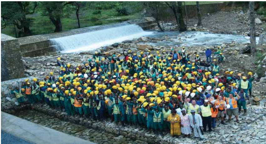
Construction work at NRE's micro-hydro Scheme
