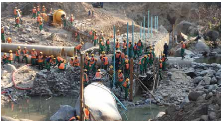
Construction work at NRE's micro-hydro Scheme
