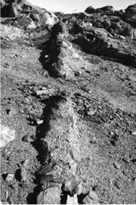
Fig. 21: During the survey in June 2022, the southern fencing of the camp was documented for the first time. It consisted of railway tracks embedded in a low cement embankment. (Photo: K. Lembke, 2022)
