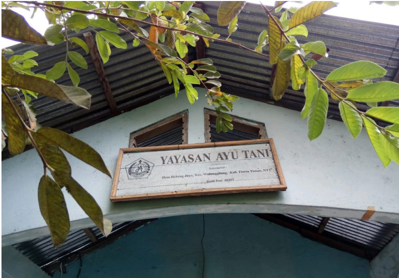
Figure 5.13. The Building of Ayu Tani Foundation
