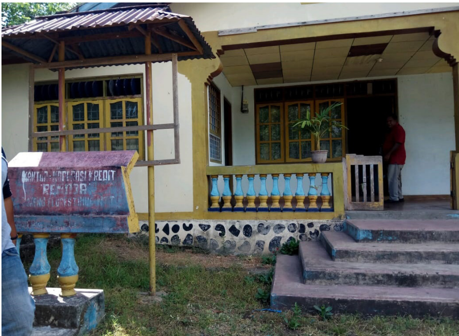
Figure 5.15. The Building of KSU Jantan
