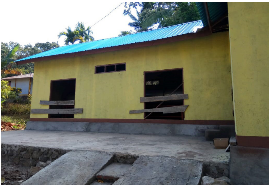
Figure 5.10. A building where The Candlenut Cracking Machine is placed
