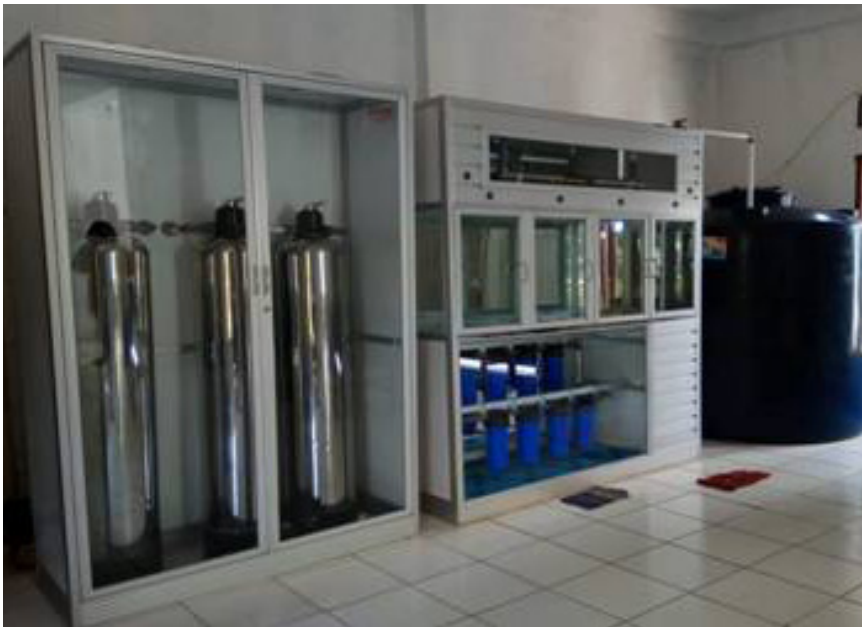
Figure 5.5. Drinking water treatment installation from springs in Boru Kedang village
