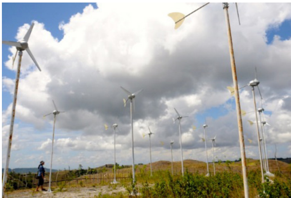
Twenty windmills in Kamanggih village in eastern Sumba Island, East Nusa Tenggara, generating 10 KW of electric power and reaching 22 households
