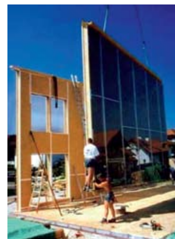
Figure 2. Assembling wall elements of a Passive House in Linz, Austria; fabrication on the spot
