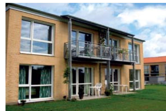
Figure 2. The Danish passive house project Rønnebækshave II in Næstved comprises a small housing block with 8 apartments realised according to the German passive house principles.
