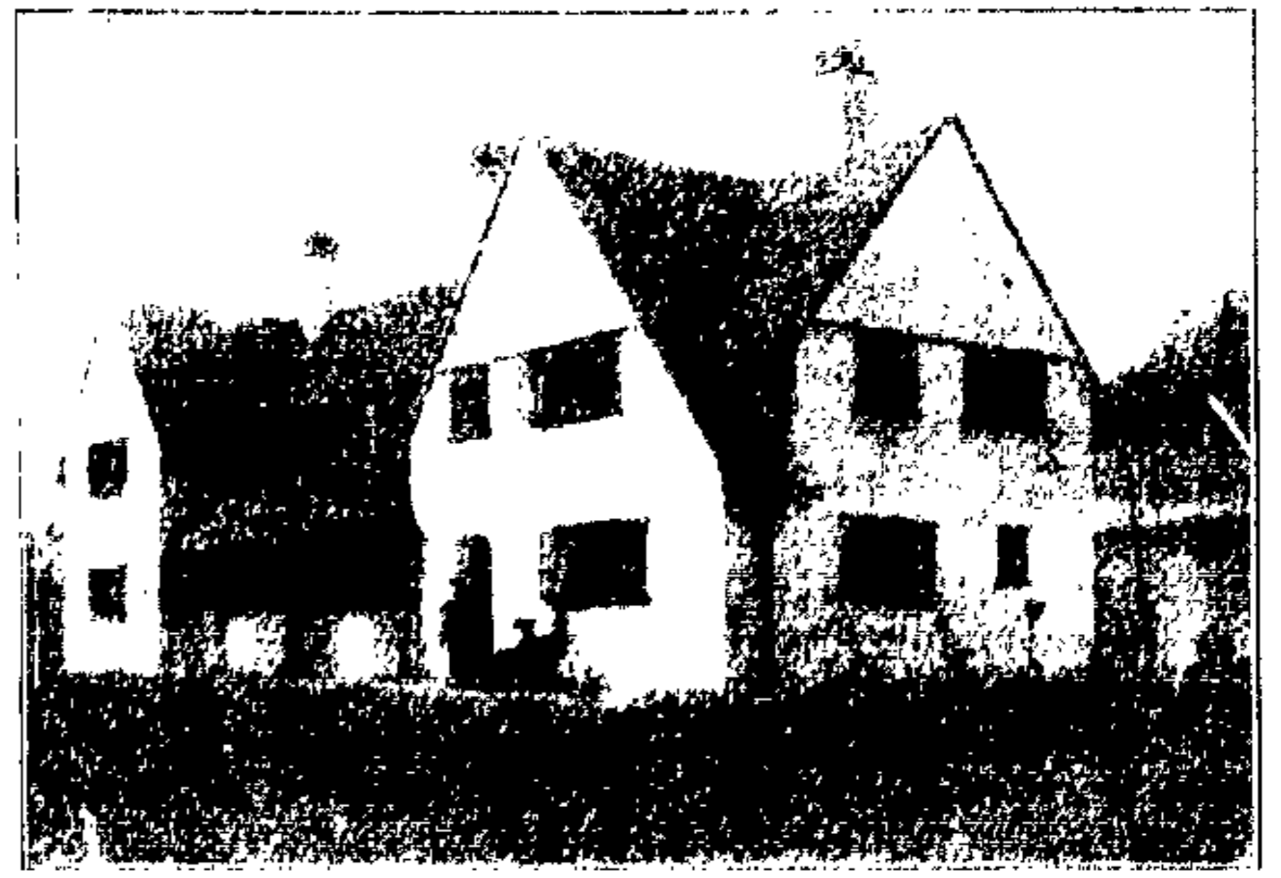
Doppelhandhaus in Leithworth.
