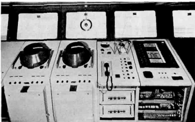
Above: Automatic bridge control of the main engines. Orders may be transmitted automatically to the main engines, thus controlling directly the speed of the propeller and the movement of the ship. Below: The engine room control console is the nerve centre of the Dolabella's entire automatic control system. (Photos: Shell)
