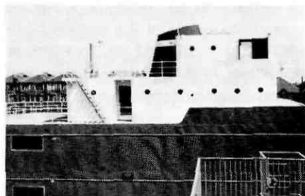
The ship built in the grounds of a British fire station to provide a training ground for shipboard firefighters.
