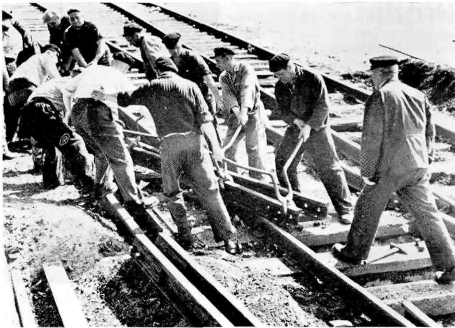
Permanent way men at work on Belgian railways.
