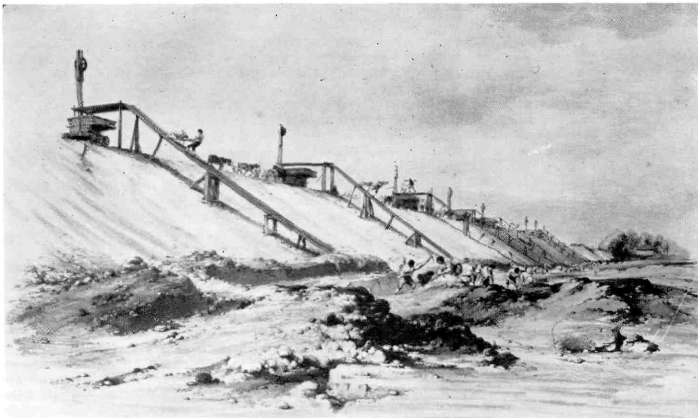
Above: Making a cutting: soil had to be lifted up the sloping walls of the cutting and dumped at the sides. A rope, attached to the full barrow and to each man's belt, ran up the side of the cutting and then round a pulley at the top, where it was attached to a horse. The horse pulled man and barrow up a narrow plank. On the downward journey the man pulled the empty barrow behind him, while the horse kept the rope taut. Below: Another early picture of navvies taking a break in their work (Radio Times-Hulton Pictures).
