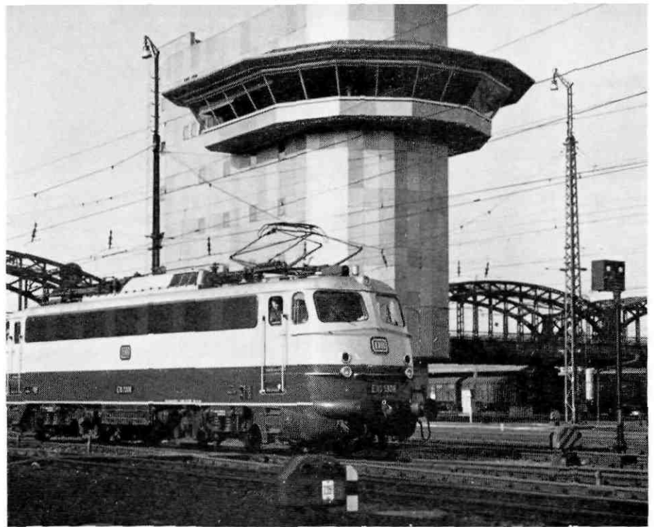
The recently constructed main control cabin at Munich Central station. The automatic equipment in use enables the train to select its own route.
