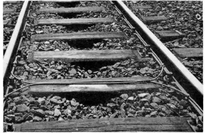
A track cable set in the rail base is a suitable means of transmitting control information to the driver's cab.
