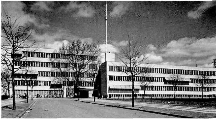
The State Broadcasting House, designed by the architect Lauritzen and built in the year 1941.
