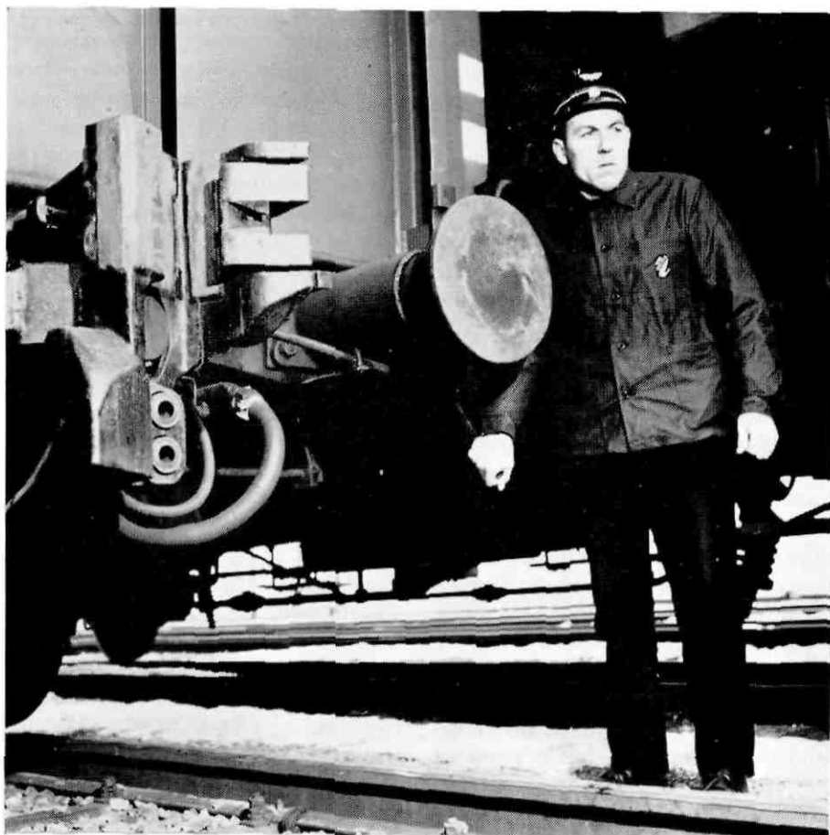
The 'Unicoupler' (Knorr), one of the rigid coupler designs accepted for testing by the UIC. This design incorporates two compressed air pipes.
