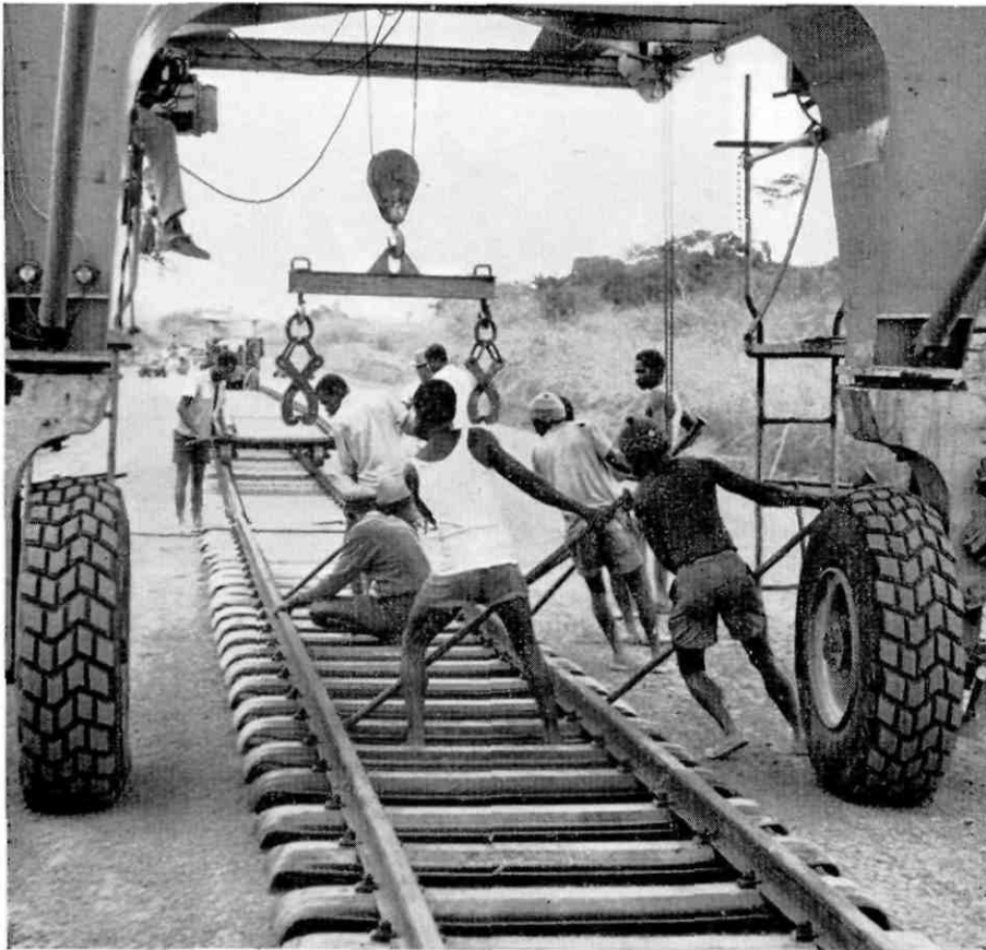
Congolese workers laying railroad track. The new African nations are intensely aware of the world spotlight on their efforts to create new forms of government (UN photo)
