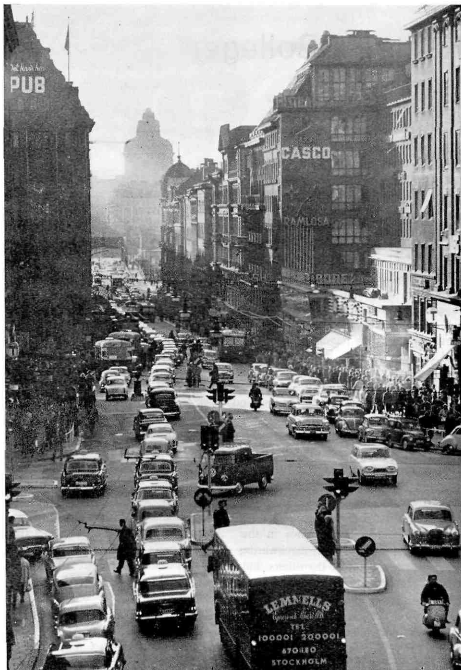
Kungsgatan, one of Stockholm's busiest streets. The city's working drivers are tired of paying fines in order that the private motorist can have unlimited space to park his vehicle.
