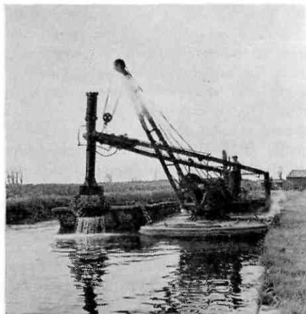
Grab dredging on the Leeds & Liverpool Canal, linking two big industrial areas (Photos courtesy British Waterways Board)
