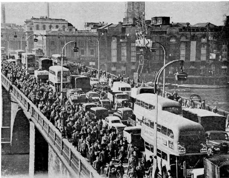
Road transport has now developed to a point where it is in danger of choking itself to death. The problem it poses in our towns must be tackled with firmness and imagination
