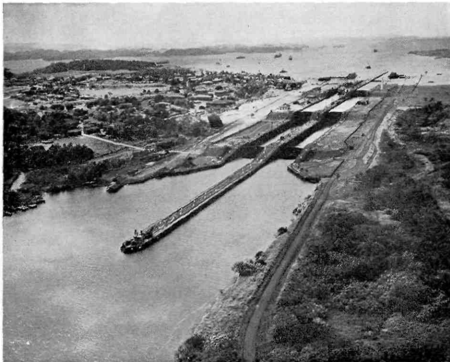
With the exception of small craft no vessel may pass through the locks under its own power. Larger vessels must be taken in tow by towing locomotives, or 'electric mules'
