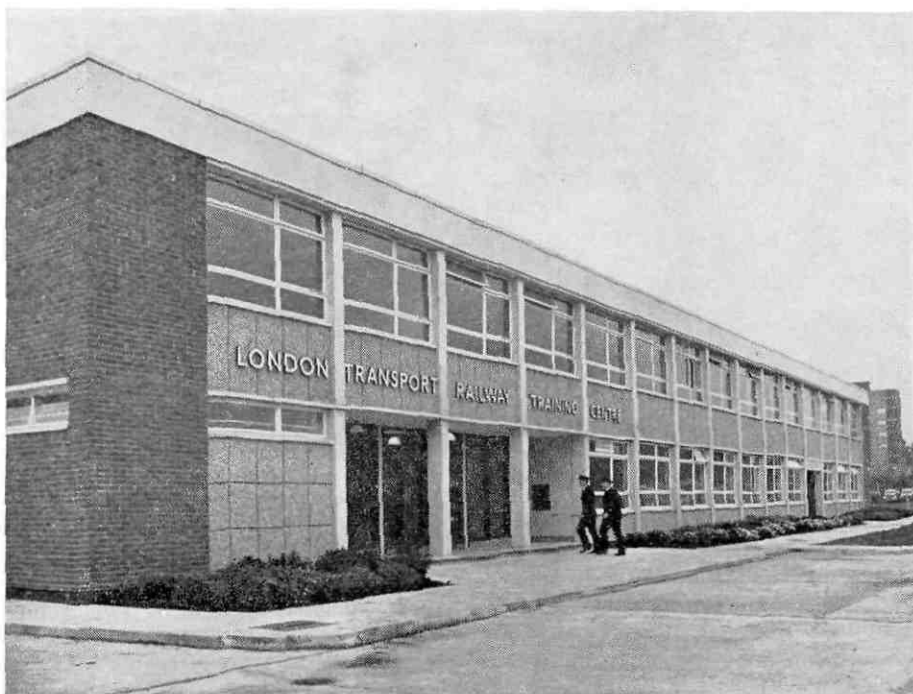
The new building for training London Transport staff at White City has clean, modern lines, and large windows have been used extensively to make the rooms light and airy
