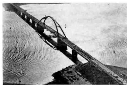
The rail-highway bridge is 'Vogelfluglinie's' major engineering feature. The new link is expected to cut international passenger train journey times between Hamburg and Copenhagen by an average of 100 minutes
