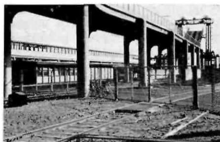
Ferry berths have elevated roadways to serve the upper decks of double-deck ferries. The 'Bee Line' entailed building 55 km of new railway track, two bridges for rail and roadways, and two new ferry terminals (photos and material reproduced by courtesy of International Railway Journal)
