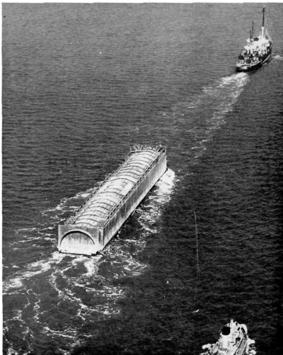
This picture shows one of the thirty-seven giant tunnel sections — each about three hundred feet long — being towed from Orange in Texas to Norfolk, Virginia, a journey of 1,700 miles. After fitting out the tunnel sections are floated to the site, positioned and sunk into a trench dug into the ocean bed
