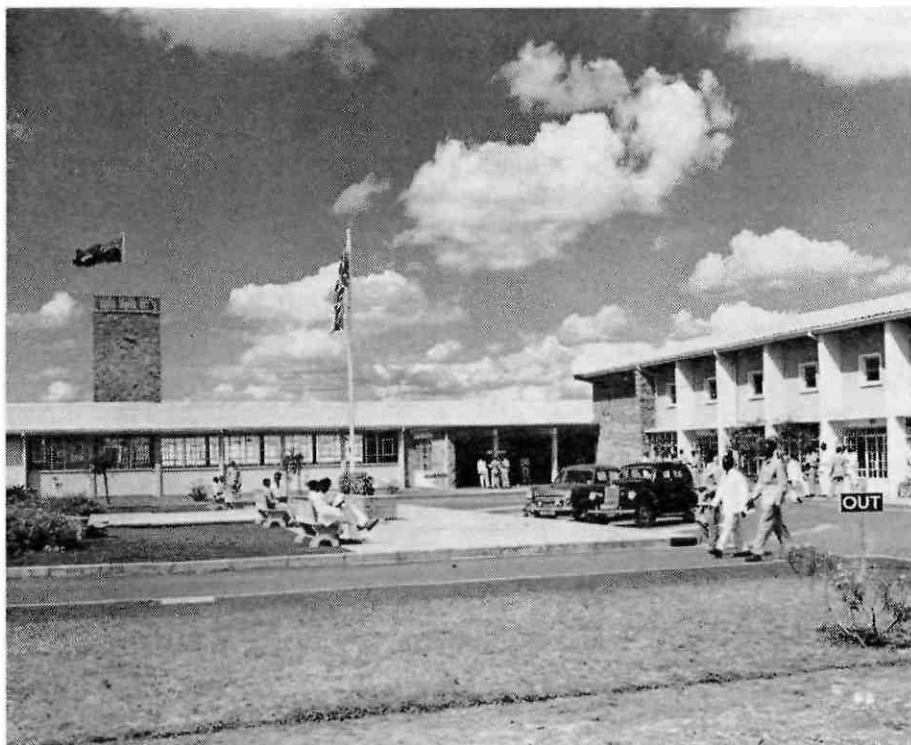
The East African Railways and Harbours Authority has three training schools of its own: two in Nairobi, Kenya, and one in Tabora, Tanganyika. In the picture is the EAR&H Railway Training School Nairobi. The school gives courses in a wide variety of railway subjects and is well equipped with classrooms and workshops. There are in addition abundant facilities for recreation and the pursuit of leisure activities (EAR&H photo)
