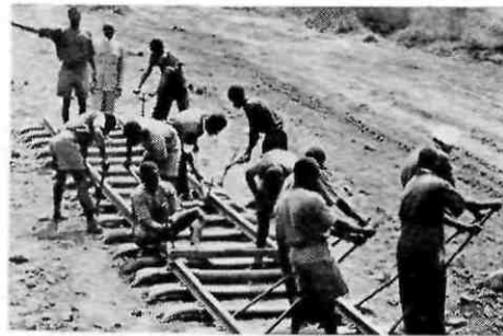
Permanent way trainees from the Nairobi Training School study track laying techniques, using special equipment available at the school itself. East African railways cover difficult and mountainous terrain and a competent permanent way staff is of immense importance to safety and smooth running (Photos from EAR&H)
