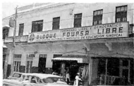
Headquarters of the democratic trade union centre in the Dominican Republic, known as FOUPSA LIBRE. The building also contains the Institute of Trade Union Education. The Dominican trade unions are making substantial progress in organization and collective bargaining since Trujillo
