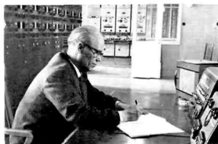
At the Helsinki radio station. On the left are some of the receivers used in teleprinter and telegraphy communications with other commercial radio stations in Europe and other continents. Through the door in the background can be seen the radio telephone terminals for communication with Hamburg and New York
