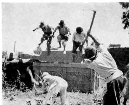
A graphic illustration of the primitive methods which are still in use in many of the more remote areas of Latin America. Andean Indians, building their homes the hard way, are here seen jumping on forms to pack the earth into solid walls
