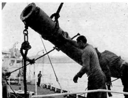
The loading of the oil at Baniyas, the Iraq Petroleum Company's pipeline terminal on the Syrian seaboard, is done off shore. Sealine gangs board the tankers and connect a flexible pipeline; a signal is given to the shore station and loading operations begin (IPC photograph)
