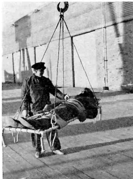
This photograph demonstrates the usefulness of stretchers slung from cranes in transporting an injured man from ship to shore. The stretcher is equipped with sturdy legs and strapped canvas bands keep the injured man secure
