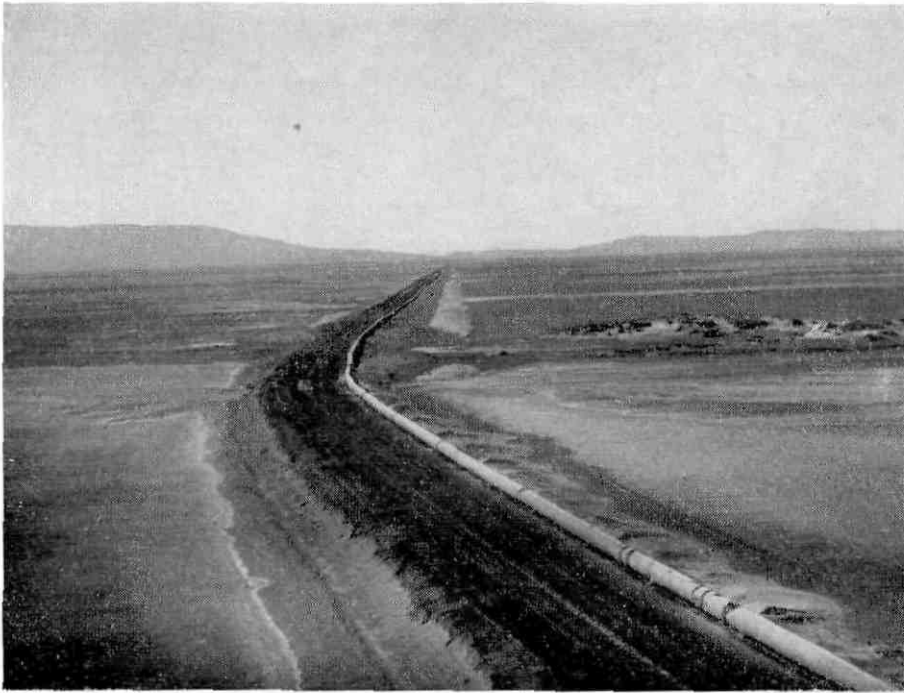
Life-blood of our highly developed mechanical civilization, oil is more frequently found in worth-while quantities in regions far removed from those areas where it finds intensive use. This Shell photo shows a pipe-line in Venezuela bringing the crude oil from the oil field down to the refinery on the coast
