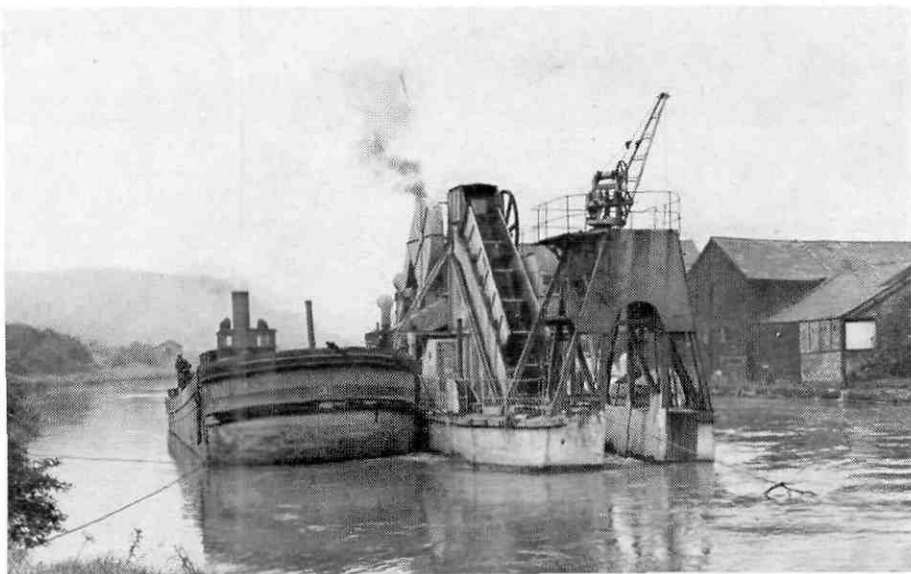
British Waterways has an ambitious development programme for the main waterways and has also stepped up its work on maintenance. Shown here is bucket dredging on the Weaver Navigation
