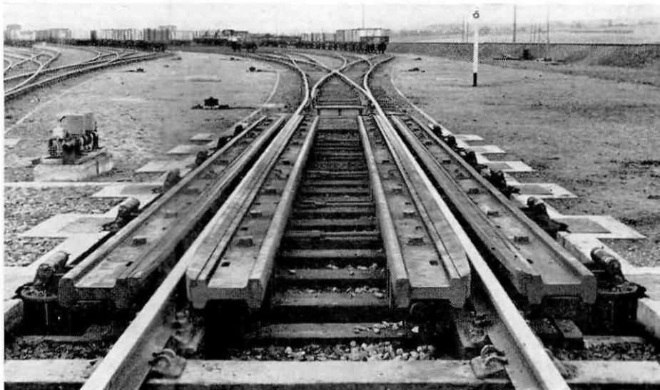
ABOVE: Beam aerial which is used in measuring the speed of approaching railway wagons BELOW: Wagon retarders grip the wheels, the force of the grip being determined by a computer
