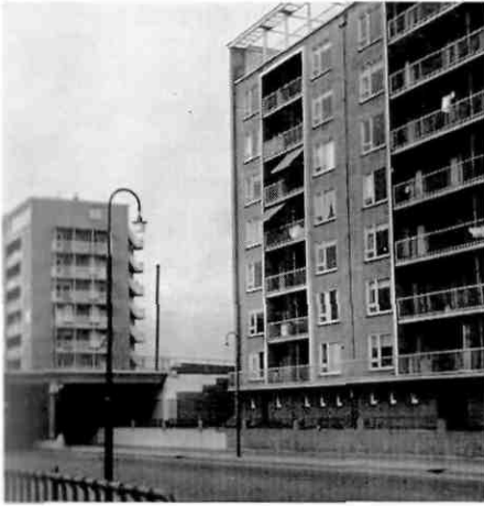
A very large amount of new housing is now to be seen in the outer suburbs of Amsterdam. These new flats are in the Western area of the city
