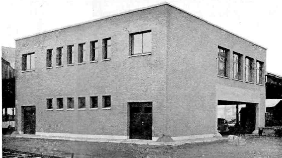
Exterior of the new dockers' canteen recently opened at the Leopold Dock in the port of Antwerp. This is one of a number of modern canteens being built in the port under a scheme started in 1956
