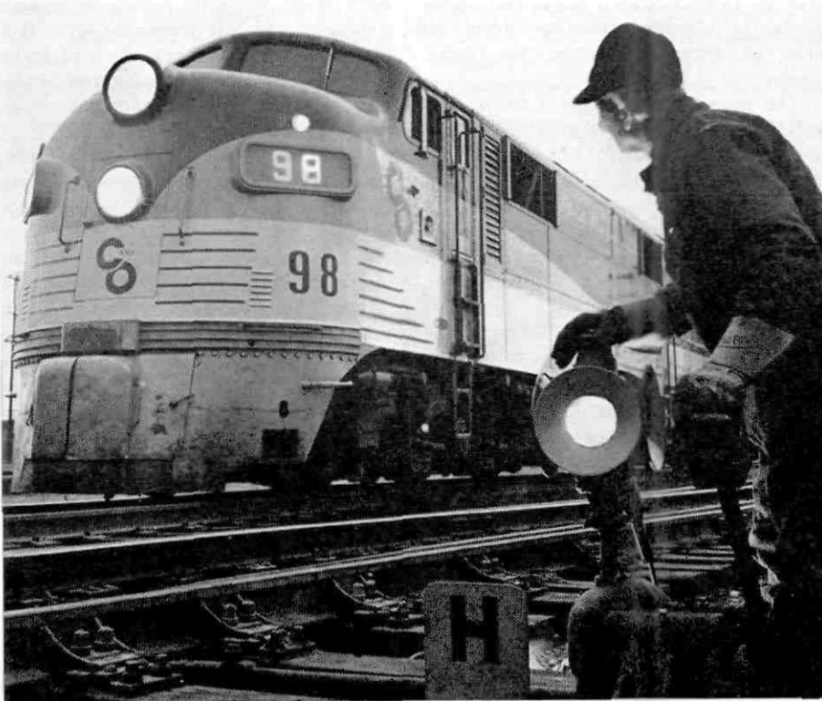
A switchman on the Chesapeake and Ohio Railway throws a switch as a modern diesel train passes (Photo by courtesy Chesapeake & Ohio)
