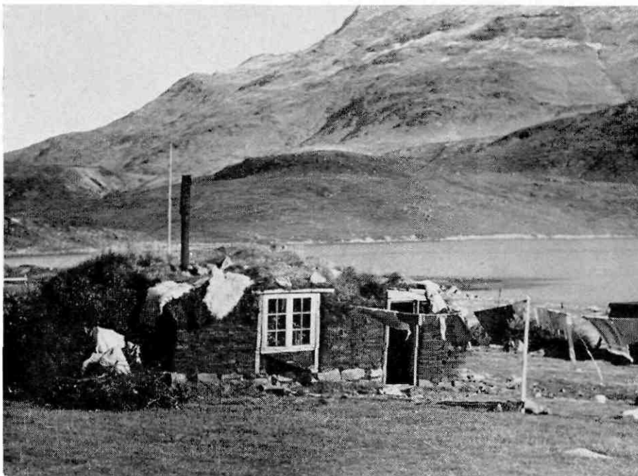
Primitive turf-huts like this are still to be seen in Greenland, especially in many smaller settlements. They are, however, very easy to keep warm
