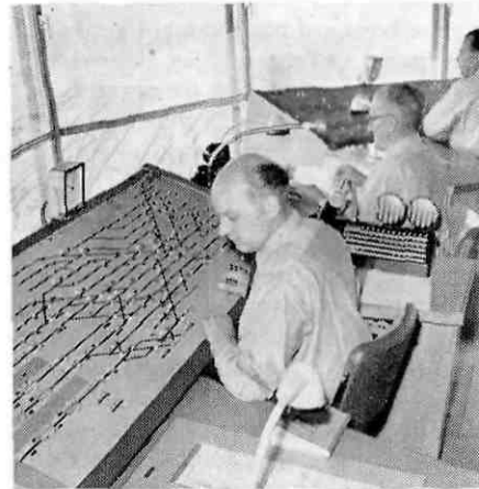
High up in the control tower at one of the five signals control panels. This operator is controlling shunting operations in the area for which he is responsible about 4,500 operations every day
