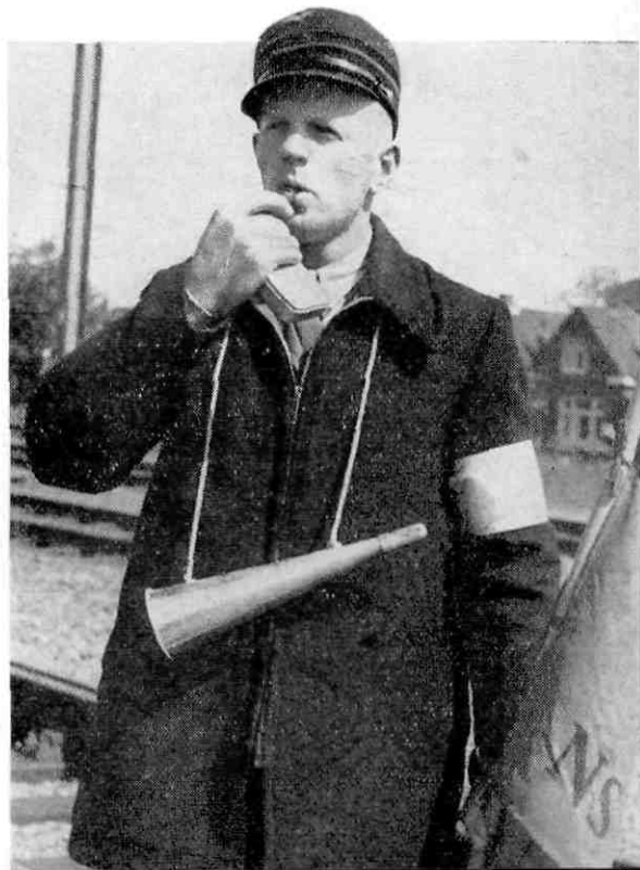
While his colleague is engaged in grinding down a point, the look-out man watches for approaching trains. When conditions are unfavourable more than one look-out is posted, of whom one stands by the gang and the others farther along the track
