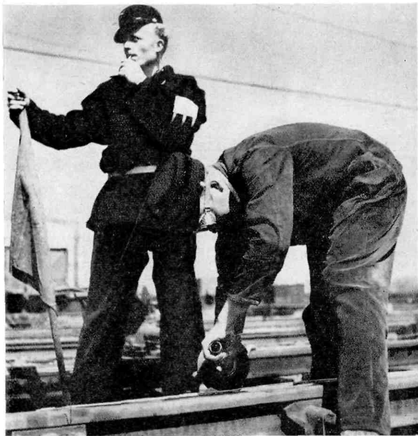
While his colleague is engaged in grinding down a point, the look-out man watches for approaching trains. When conditions are unfavourable more than one look-out is posted, of whom one stands by the gang and the others farther along the track
