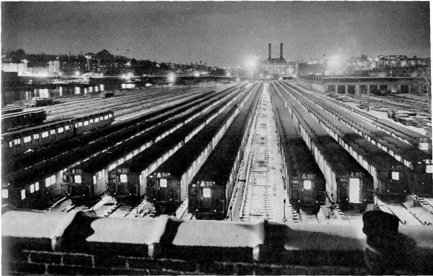
The 207th Street inspection yard. This scene, taken on a winter night, reflects the vastness of subway operation in New York
