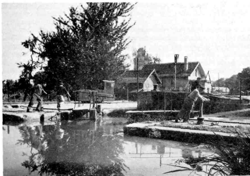
Apart from a few showpieces, such as those on the Paris-Le Havre Canal, the vast majority of locks on the French inland waterways are still worked by hand. A number of canals date back to the time of Henri IV and many are falling into disrepair. Notable exceptions are the Canal du Nord and the Saint-Quentin Canal.
