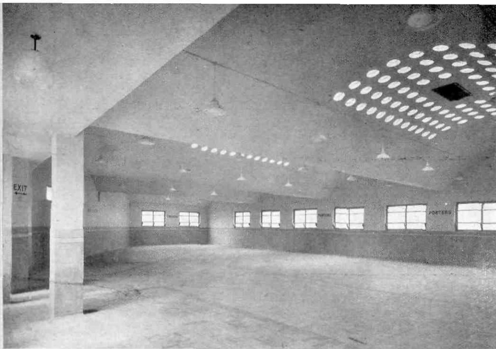
British dockers no longer have to wait around for work in all weathers. Our photograph shows a modern call stand built by the National Dock Labour Board
