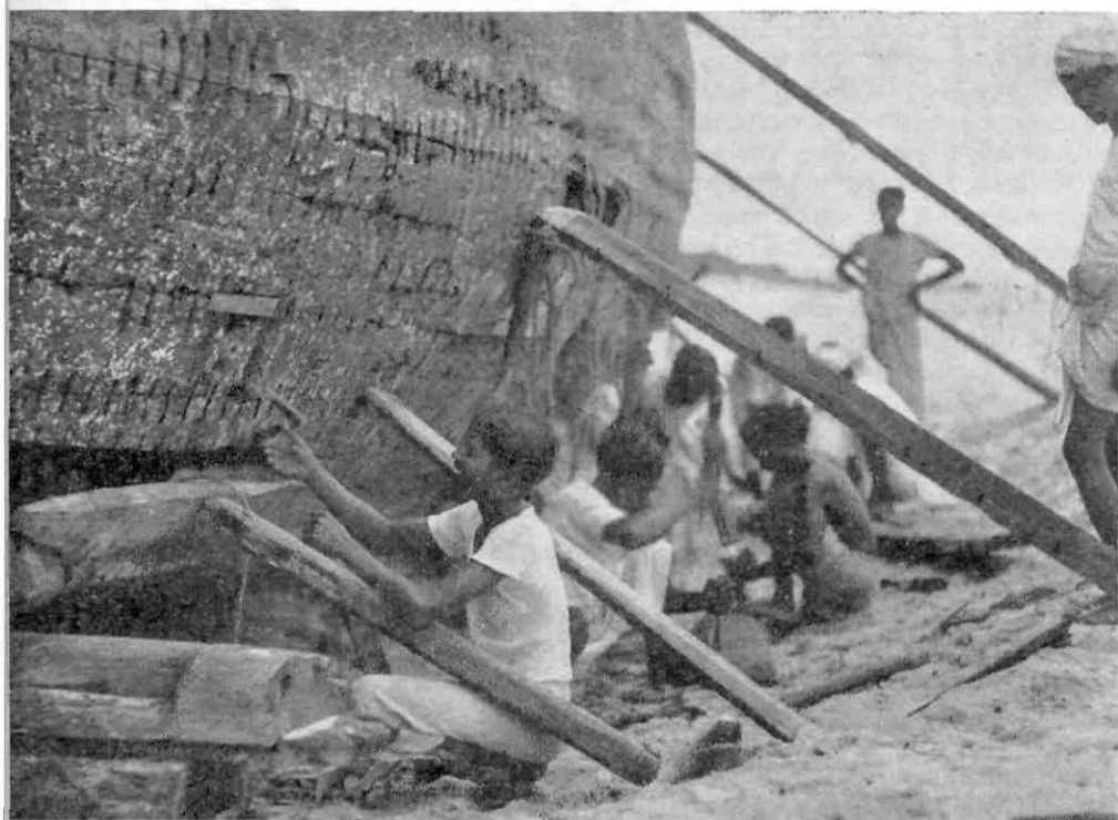
Fishermen from Cochin are here seen repairing one of their craft. The Norwegian aid team found that fishing boats in this region are both sturdy and well-built
