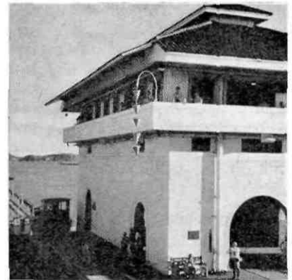
As the 'Caronia' leaves the east chamber, the five-cone signal on side of house at Pedro Miguel Locks indicates that the vessel required ten 'mules' or locomotives.
