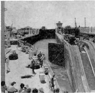
S.S. 'Caronia' entering lower chamber of Gatun Locks. The gates are just opening. Passing through the lock, the vessel will be raised eighty-five feet above sea level.
